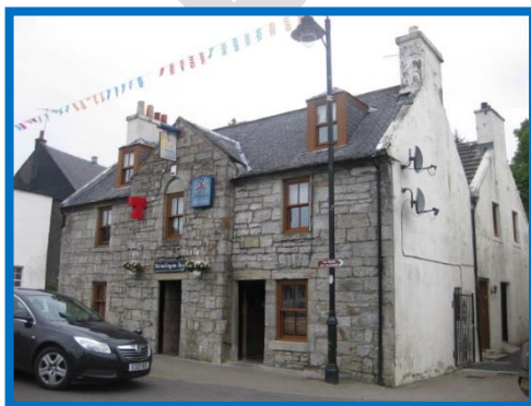
Figure 9 The Dalmellington Inn formerly the Railway Inn
