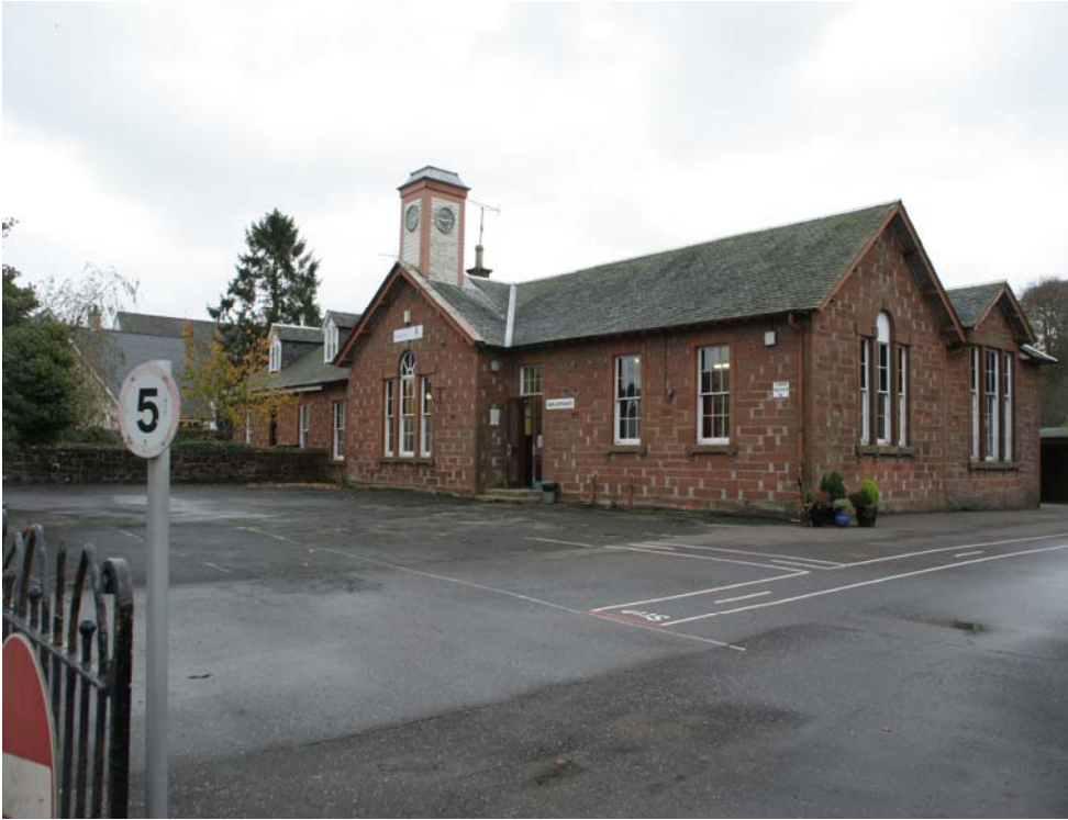
Photograph 1 : Front elevation from the entrance gate
