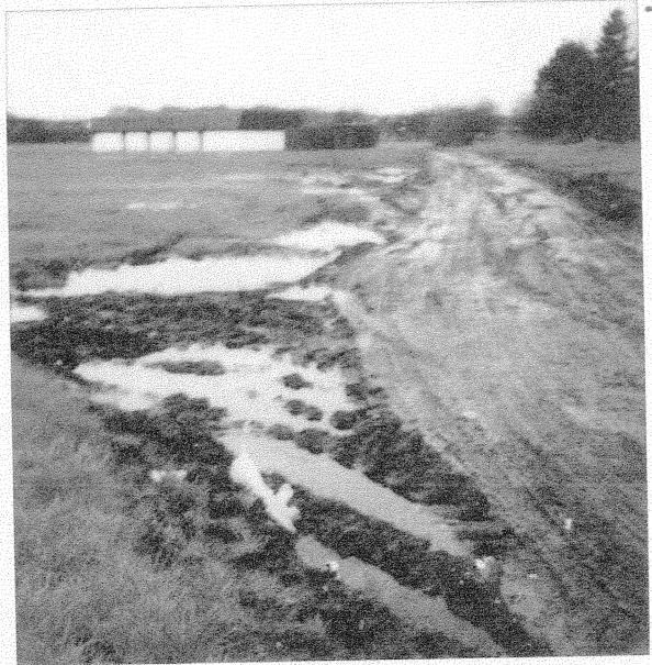
Dec 04 - Quagmire conditions at the New Mill Rd entrance
