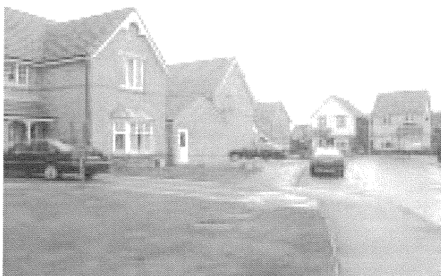
Allocated and Unallocated Car Parking Spaces
