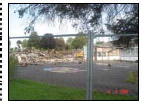
Demolition of Park School
