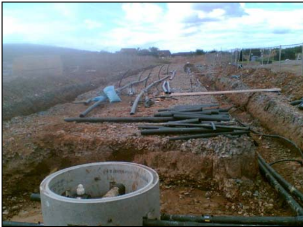
Ground Source Heating being fitted – 3 August 2007
