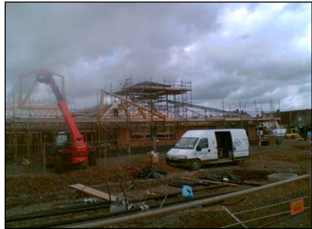
Work on external walls & roof ongoing – 3 August 2007
