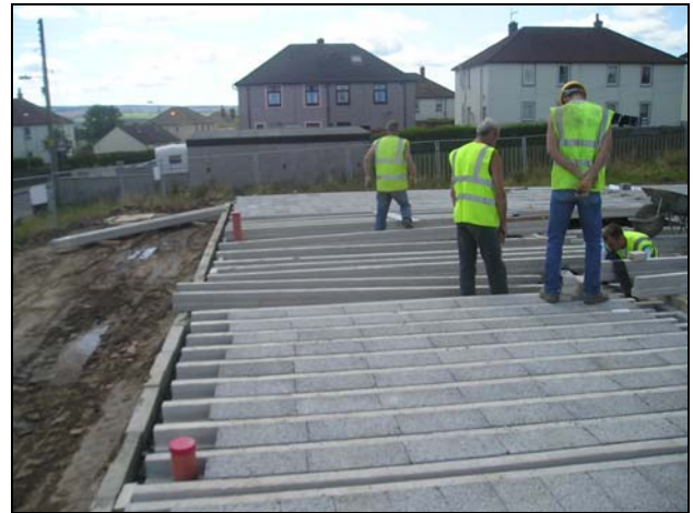
Suspended concrete floor (B) – 09-08-07
