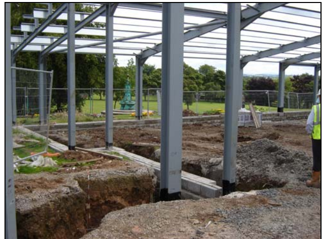
Works to Substructure – 13-08-07
