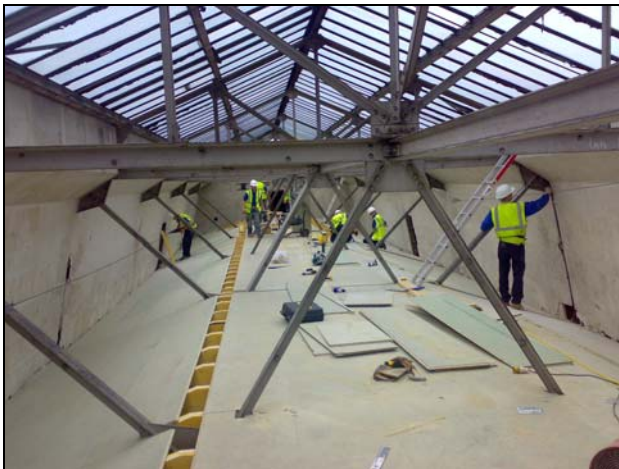
Internal roof works (1) – 13-08-07
