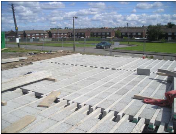
Suspended concrete floor (A) – 9-08-07
