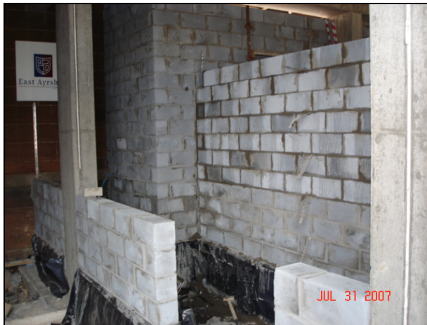
Internal blockwork – 31-07-07
