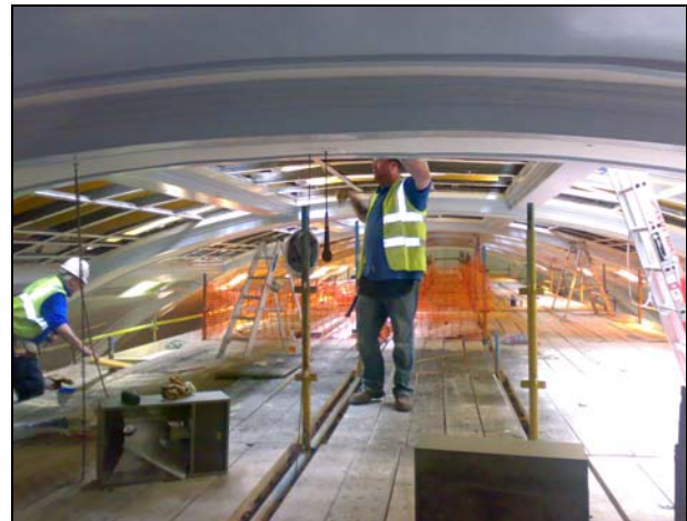
Internal Roof Works (2) – 13-08-07
