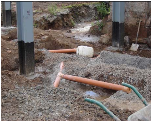
Works to Drainage (1) – 13-08-07
