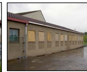
External View – July 2008
