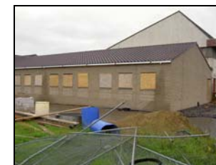
External View – July 2008
