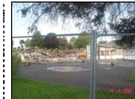
Demolition of Park School
