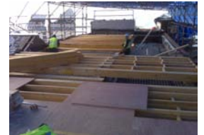
New Timber Joist
