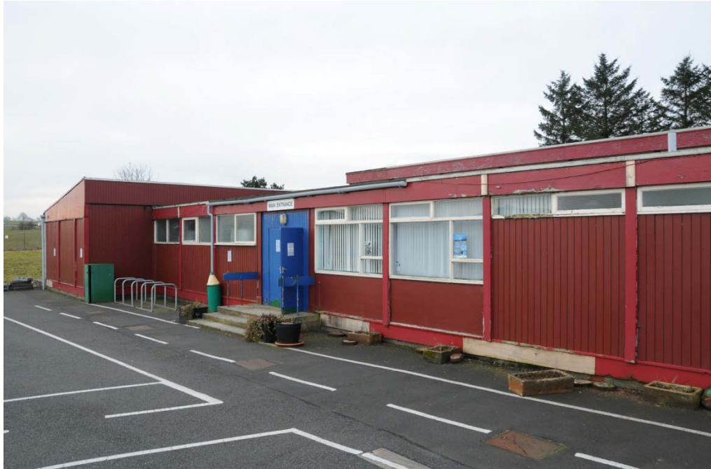
Photograph 1 : Front elevation from the playground.
