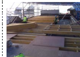
New Timber Joist
