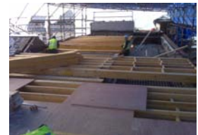
New Timber Joist
