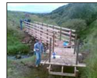
Footbridge at Loudoun Hill
