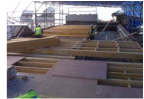
New Timber Joist
