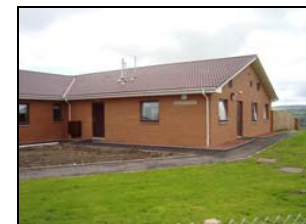
External View – July 2008
