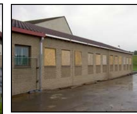
External View – July 2008
