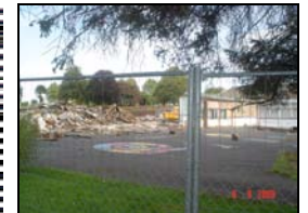
Demolition of Park School
