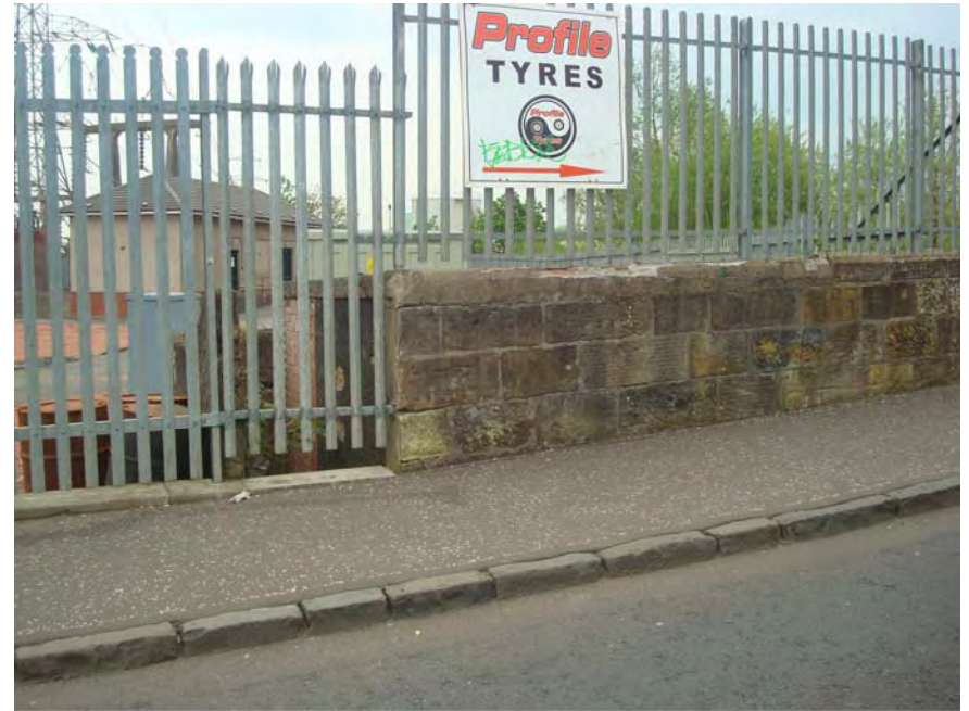
Former Public Conveniences – Old Street - Kilmanrock
