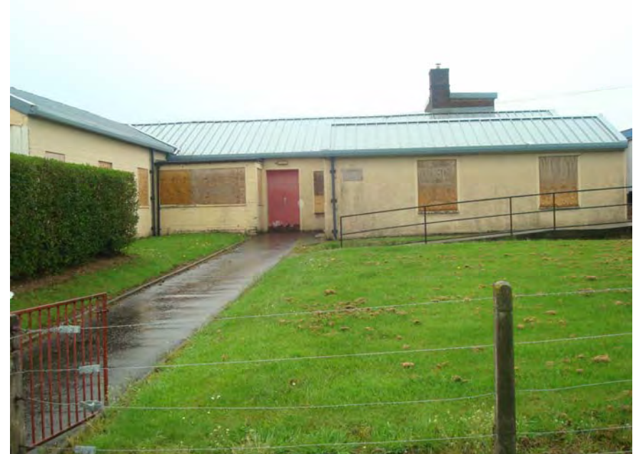
Former Hillbank Nursery (Main Building) – Hill Street - Kilmarnock
