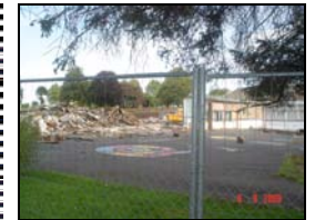
Demolition of Park School
