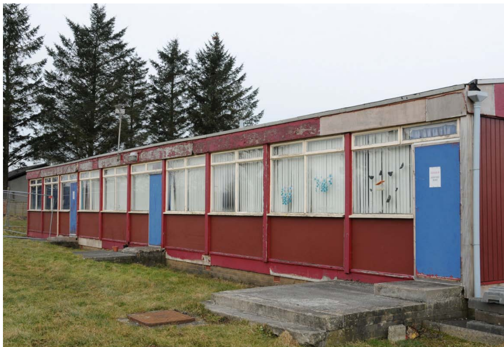
Photograph 4 : External view of east elevation. The corner timber post at the far right of the photograph was replaced in 2009.
