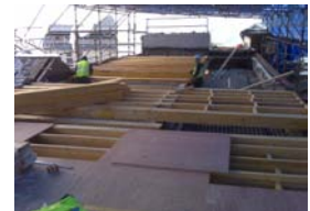
New Timber Joist
