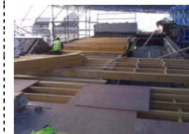
New Timber Joist
